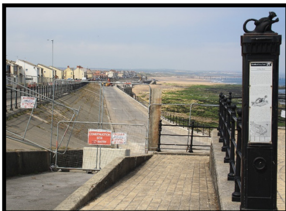
No access along Sea View Terrace due to construction works (/C0303C02)
