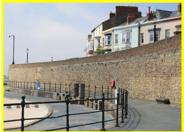
Rear masonry wall in fair condition (/C0401C04)
