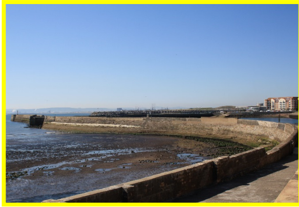
North face of North Pier (/C0401C22)
