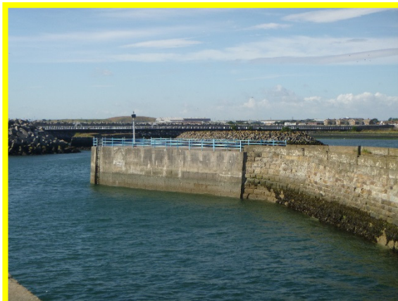
Head of inner arm of North Pier (/C0401C21)
