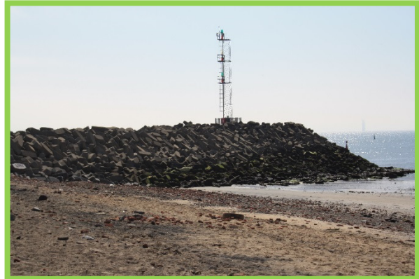
Middleton Jetty south aspect (/C0401C16)
