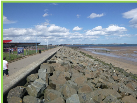
Rock armour revetment and concrete seawall (/C0401C33)
