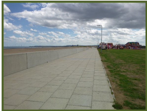
Promenade looking south towards pumping station (/C0501C02)
