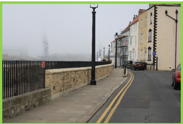
Recently completed masonry wall and walkway to rear of seawall along Northgate. (/C0401C35)
