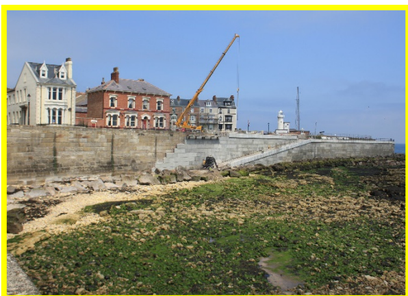
Ongoing encasement works north of Heugh Breakwater (/C0303C04)
