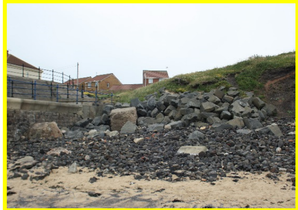
Rock armour revetment at Marine Drive seawall (/C0302C03)
