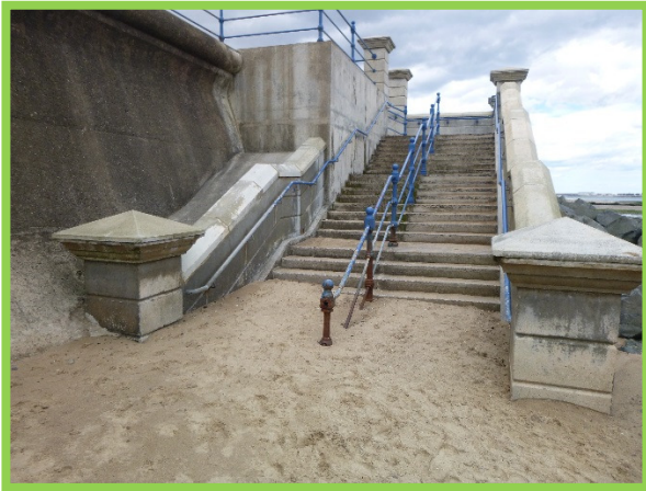
Northern access steps (/C0501C05)
