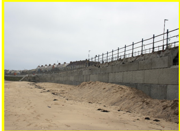
Ongoing construction of seawall encasement works along Marine Drive (/C0303C01)
