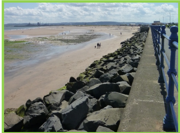
View looking south (/C0501C05)
