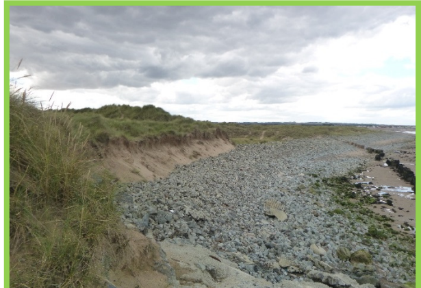
Cliffing at southern extent of dunes (/C0502C01)
