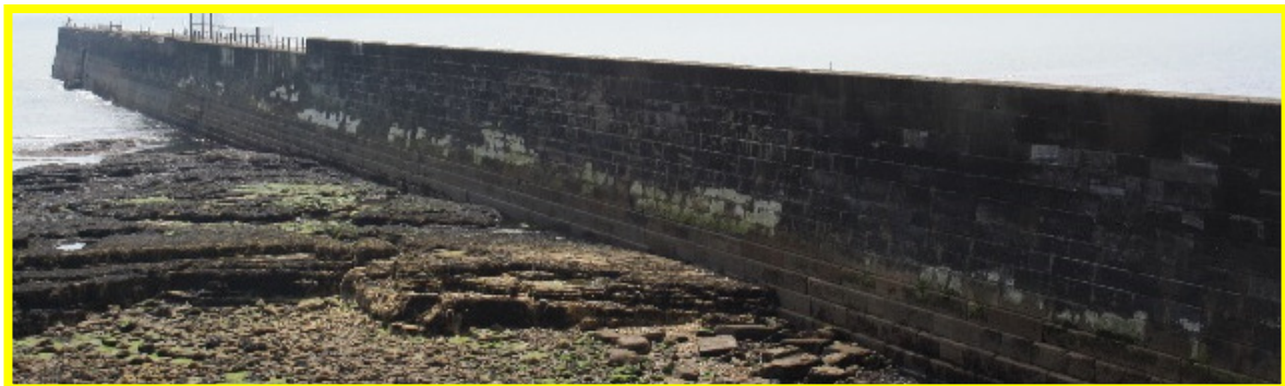
Heugh Breakwater - North aspect (/C0401C01)
