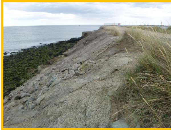
North face of North Gare breakwater. (/C0503C01)
