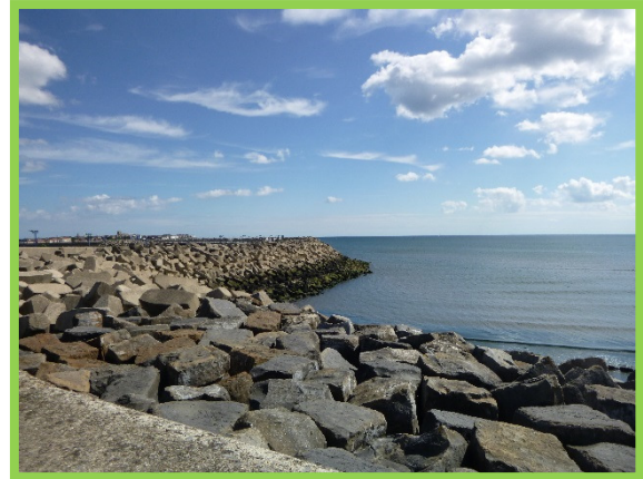
Outer face of South Pier (/C0401C32)
