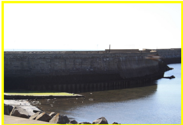
South face of North Pier (/C0401C22)
