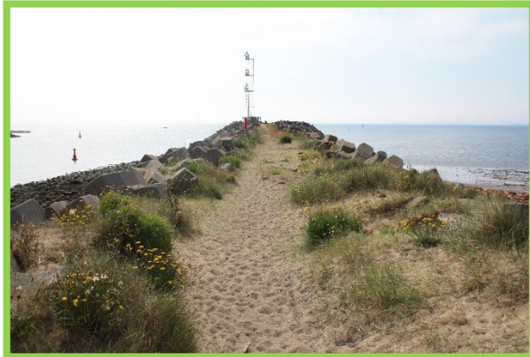
Middleton Jetty north aspect (/C0401C16)
