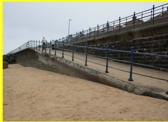
Repaired access ramp at northern end of Marine Drive (/C0303C01)
