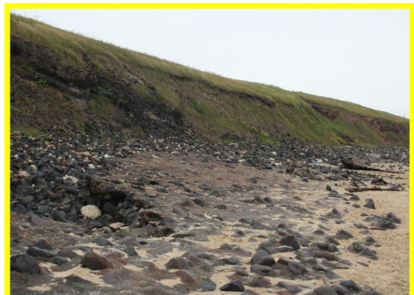
Oversteepened coastal slope, slag apron breaking up (/C0302C03)
