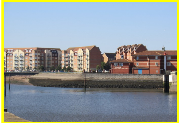
Concrete blockwork revetment obscured by vegetation (/C0401C25)
