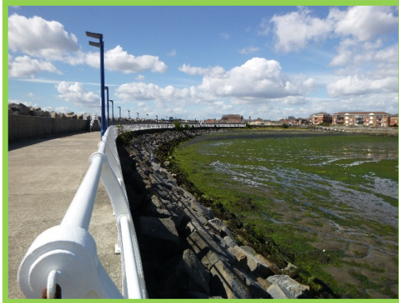
Inner face of South Pier (/C0401C32)
