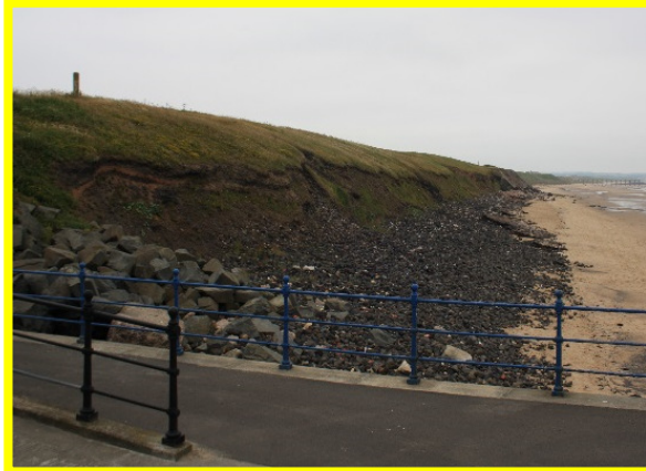
View looking north from Marine Drive (/C0302C03)
