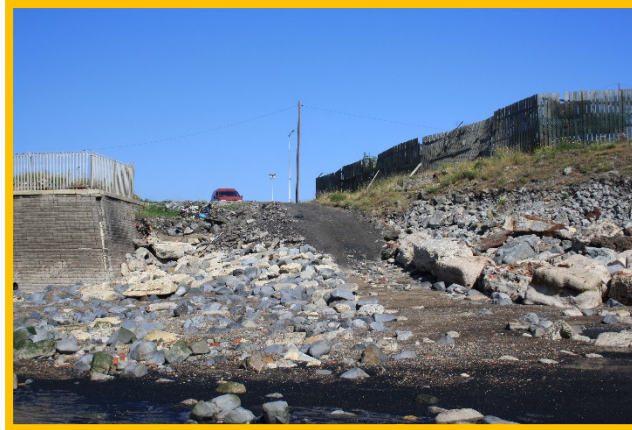
Informal access ramp (/C0401C18)
